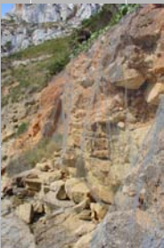
Acantilado inestable (Granadella)
